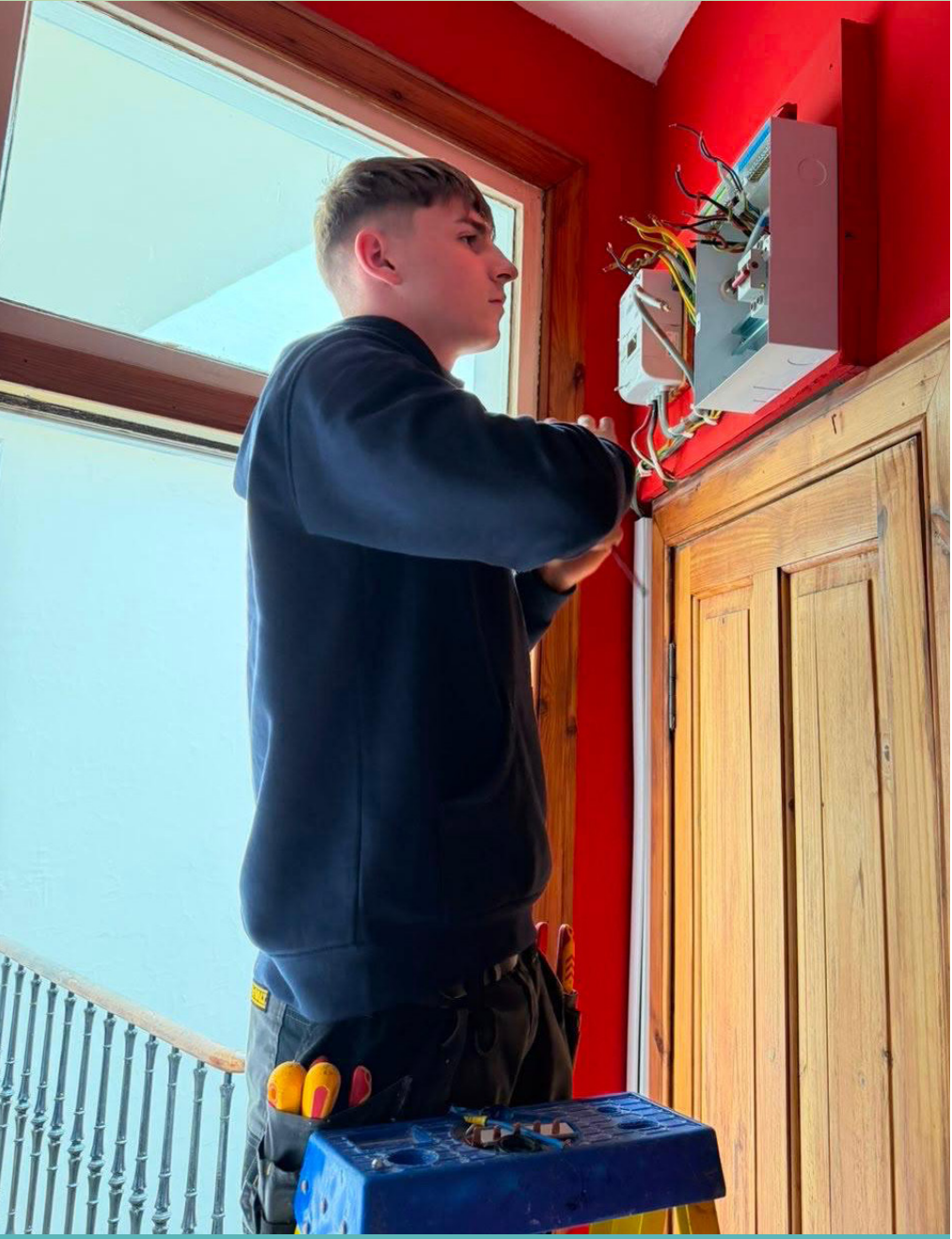
Sam at work after completing the Construction Academy
