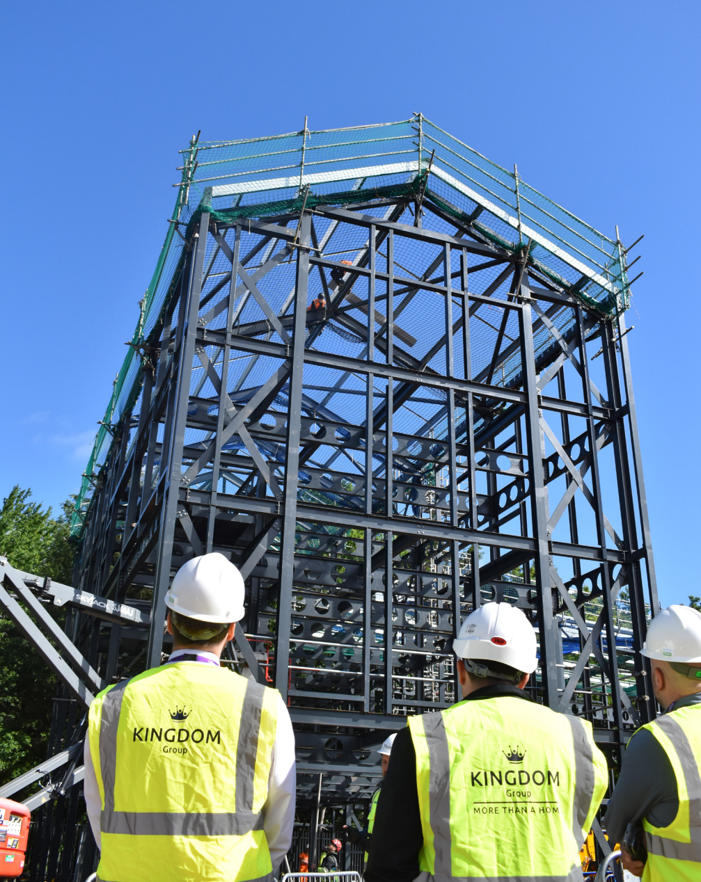
Kingdom staff visiting our new purpose built facility on Boston Road while under construction
