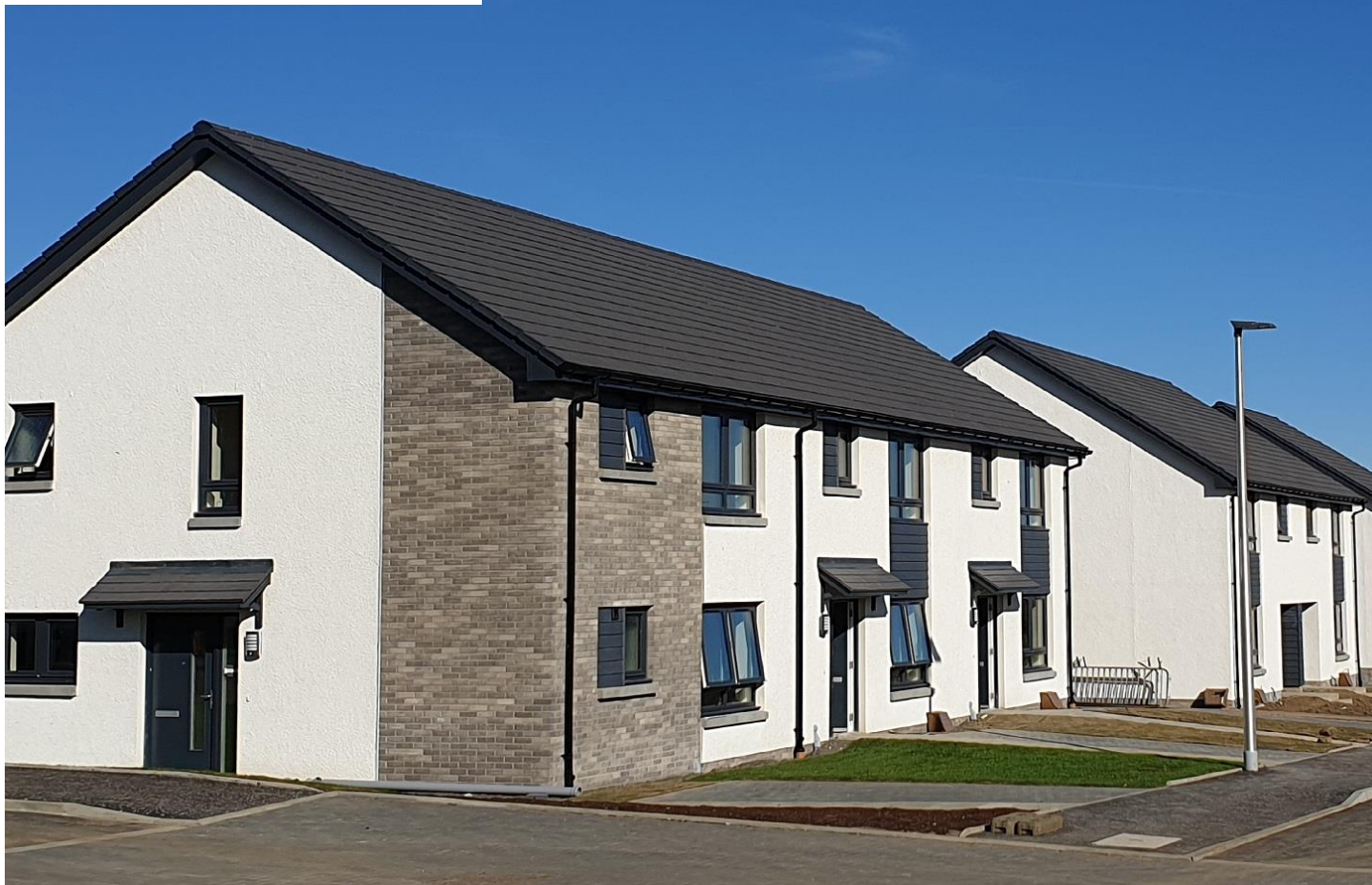
Completed Houses – Phase 1
